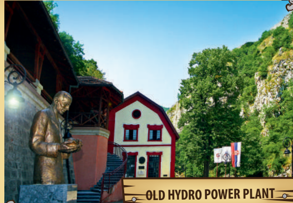
OLD HYDRO POWER PLANT
